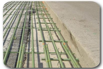
Continuously Reinforced Concrete Pavement (CRCP)
